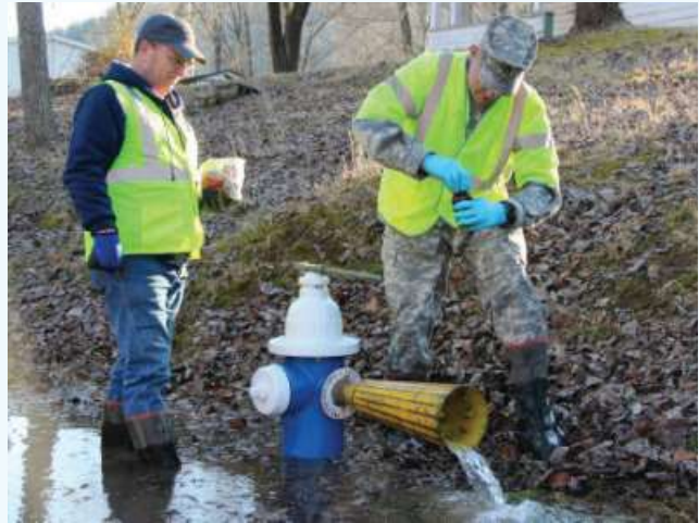
Picture 2.5: Water inspection
